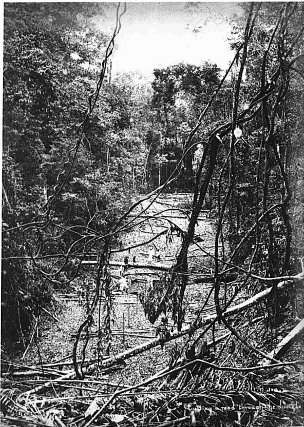
Plate 64 Cutting a road through the jungle, ca. 1890
